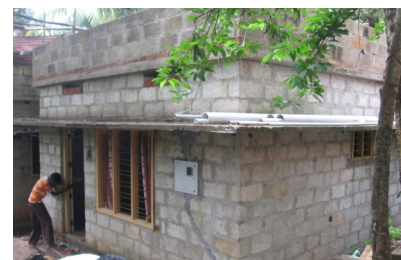
2009 Beneficiary Rajan's house after fixing the roof and walls
